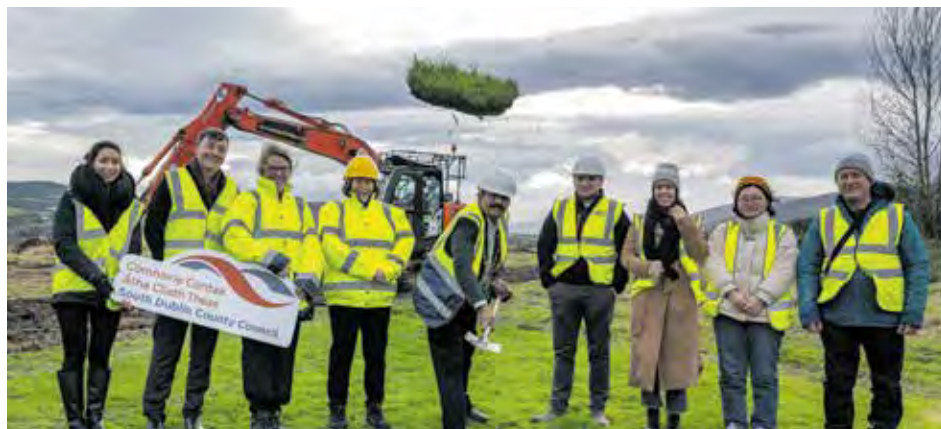
Pictured Mayor of SDCC Cllr. Baby Pereppadan with Teresa Walsh (SDCC Director of Service, Suzanne Furlong, Sean Redmond, Keith (Tim Austen Design), Shea McElhatton (ACS Civils Ltd) & SDCC staff at the sod turning for the Phase 2 works in Kiltipper Park. Pic credit: Ben Ryan
